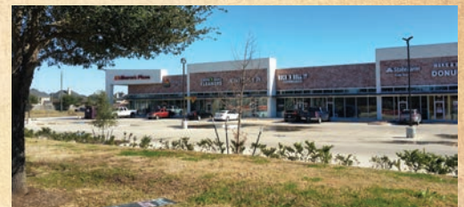
River Park West Commercial property
