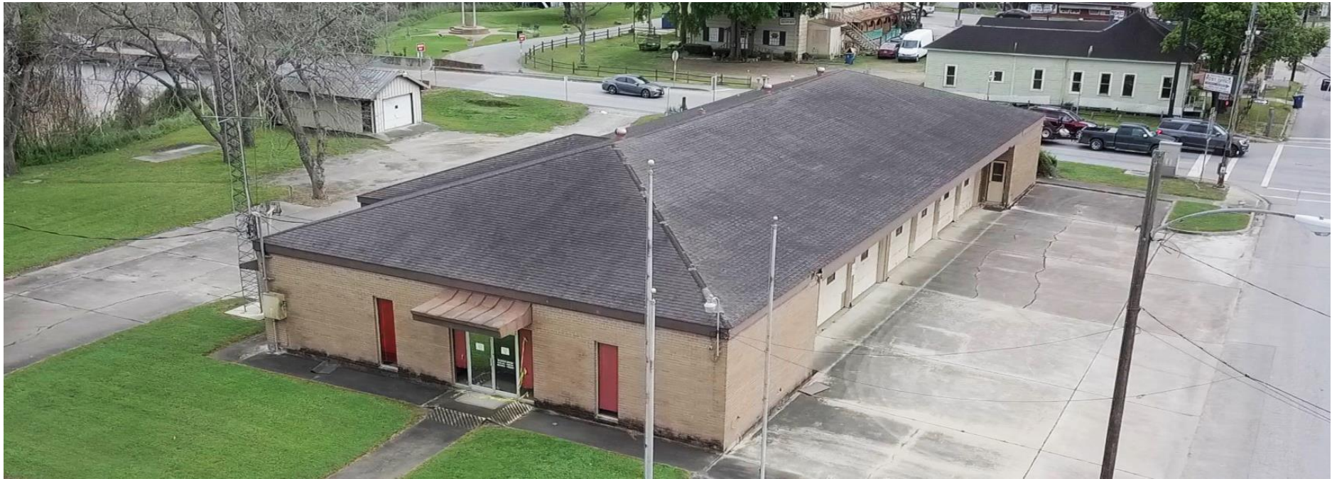
Low Roof Slope with Residential Shingles
