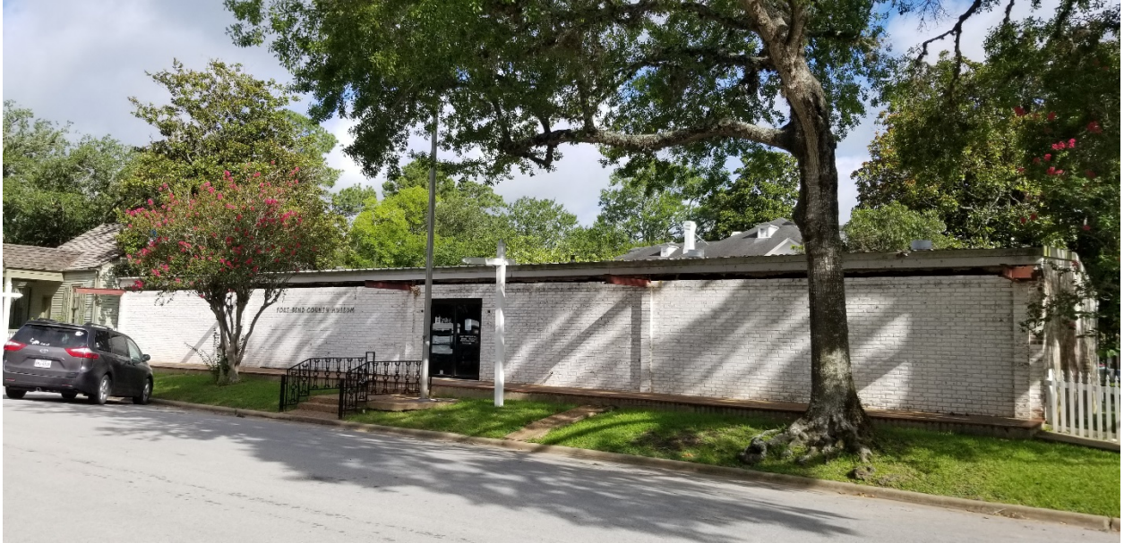
EXISTING MUSEUM BUILDING ALONG HOUSTON ST.
