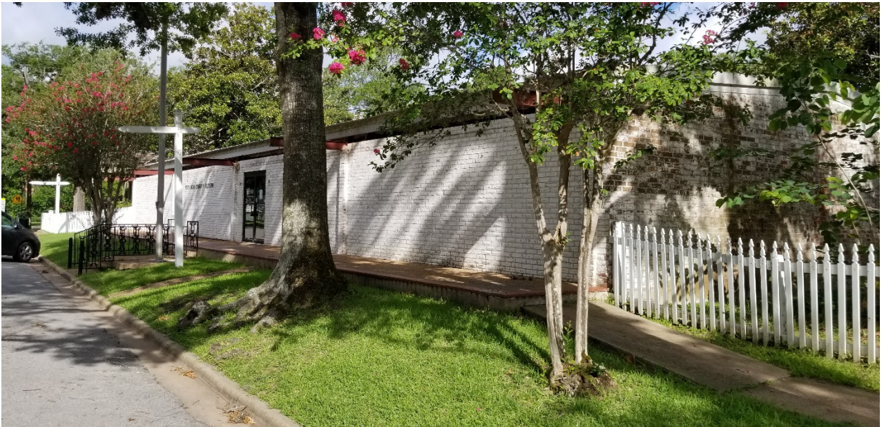
SUBJECT SITE: BUILDING WALKWAY CONNECTED TO THE SIDEWALK.
