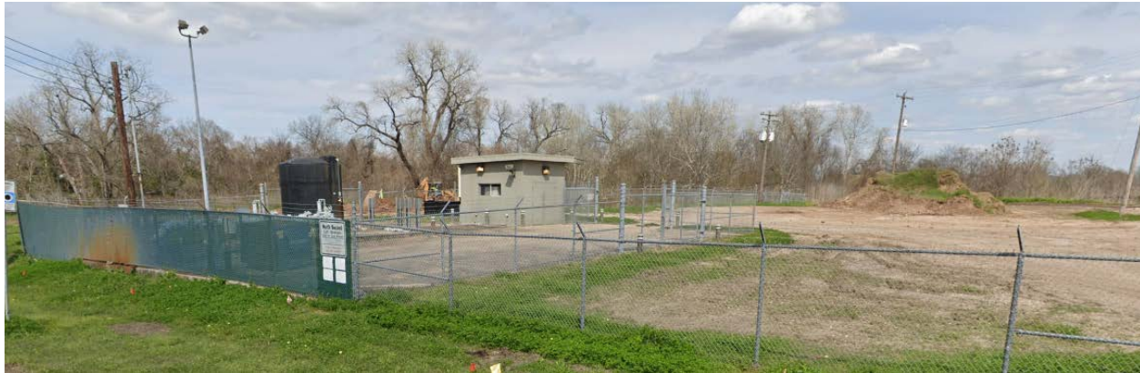
Fence Prior to the Improvement.
