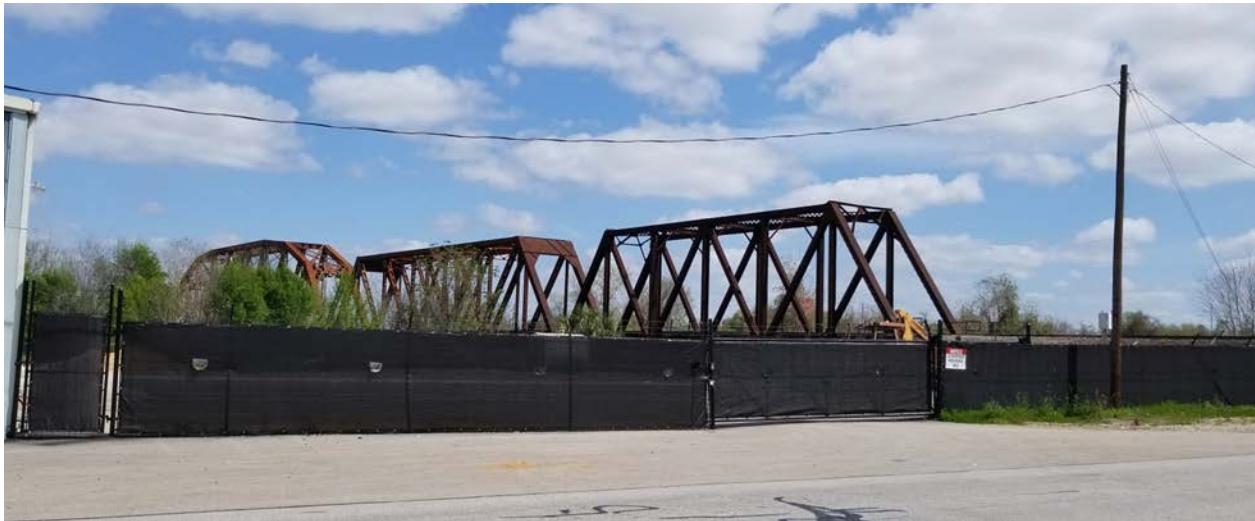
Fence after Improvement.
