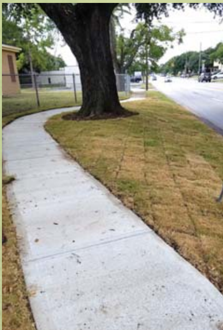
Repaired sidewalk along Jane Long Elementary School campus on Main Street
