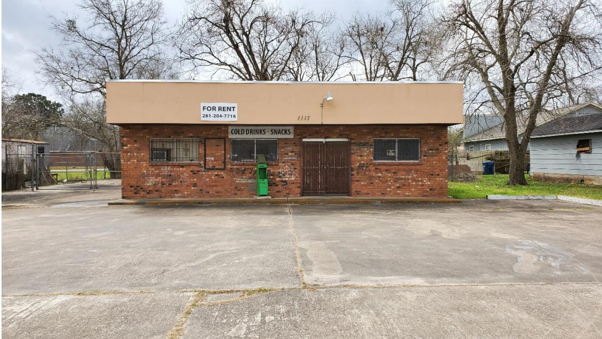
Existing Non-residential Cinder Block Building front facade
