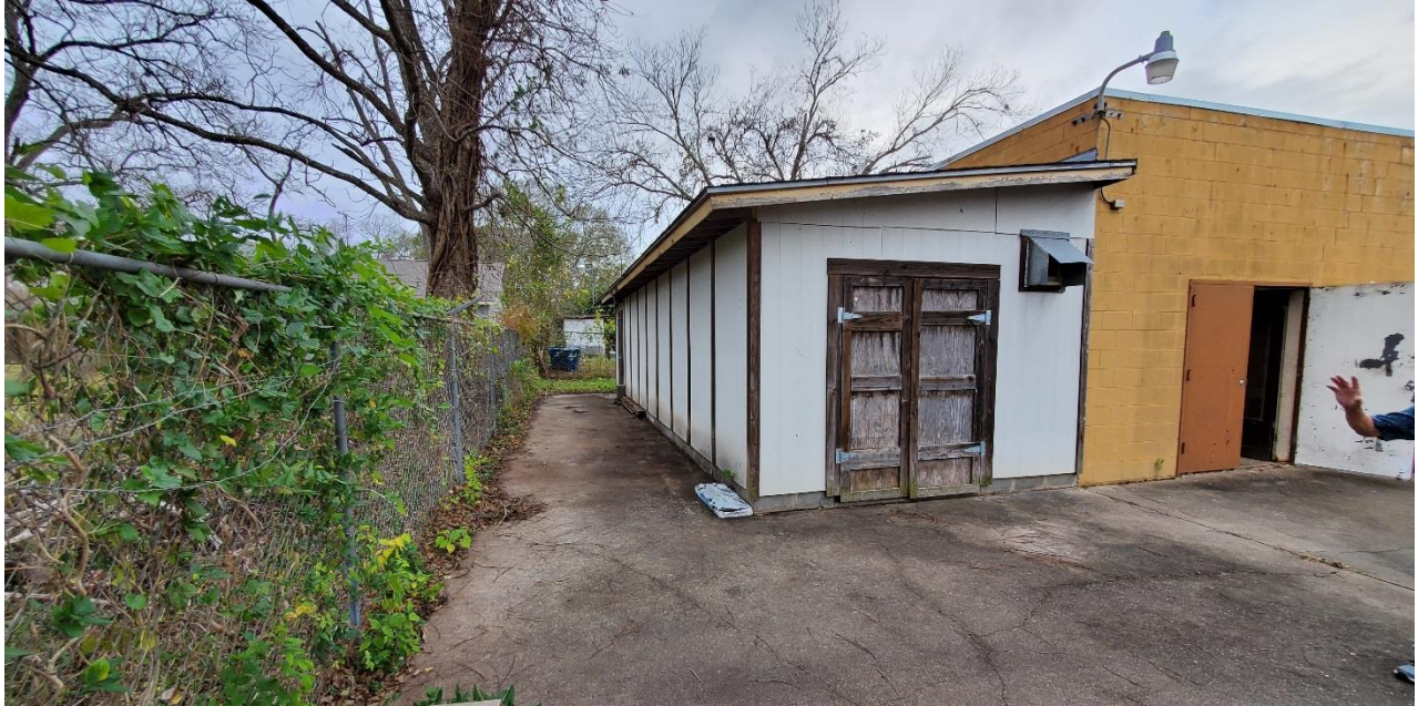
Building Exterior (Rear)
