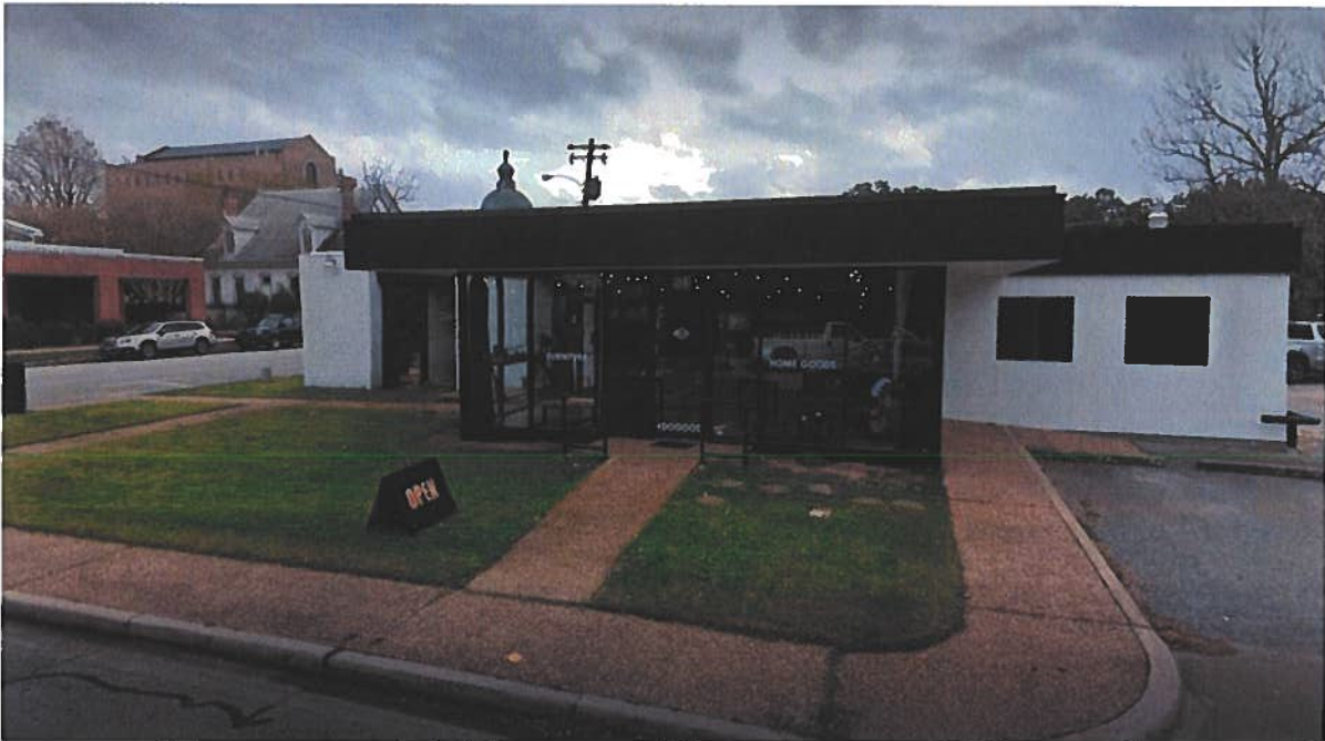
Front view of the Mercy Goods Building.
