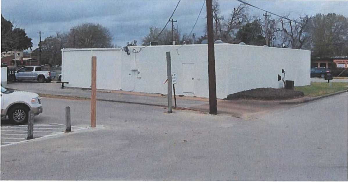
A View of the Rear and Street Side of the Mercy Goods Building.
