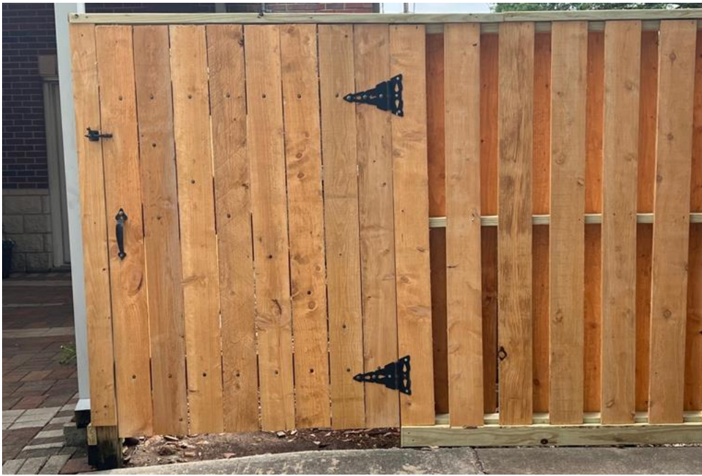
Fencing facing west towards 7 th St.
