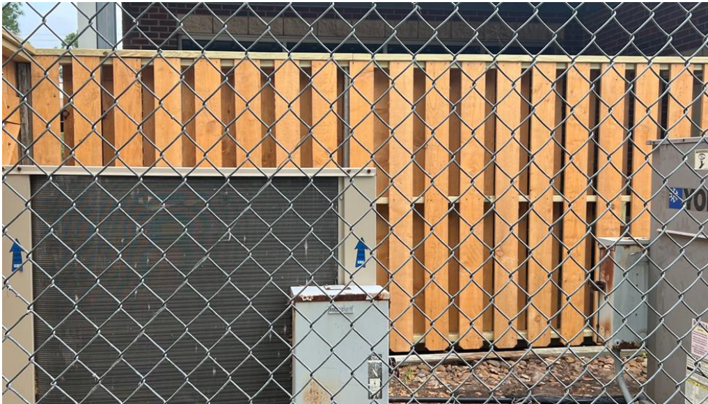
Fencing facing south towards Morton St.
