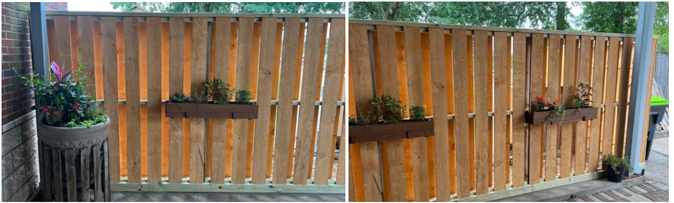
Fencing near Employee entrance facing Calhoun St.
