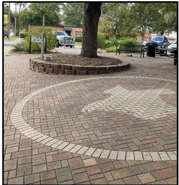
Figure 6 - Patterns Of Existing Brick Pavers May Be Continued In Newly Bricked Areas To Establish Continuity.
