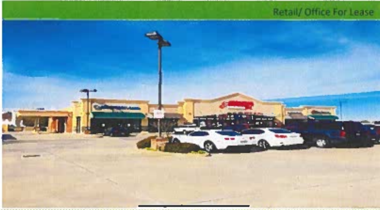
Pecan Grove Crossing 2035 FM 359 Richmond, TX 77406
