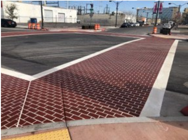
Crosswalks that contrast in color and texture from the main pavement surface can alert drivers and help slow traffic without changing the street dimensions. These, along with pedestrian warning signals, should be introduced in select locations along U.S. 90A in consultation with the Texas Department of Transportation (TxDOT).
