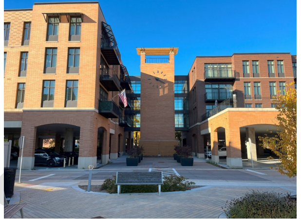
Example of “air rights” development on publicly-owned site with shared public/private parking at ground level. Podium-style construction also protects residential units from flood risk.
