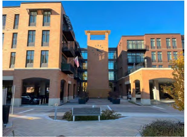
Example of private development on a publicly-owned site with shared public/private parking at ground level. Podium-style construction also protects residential units from flood risk.
