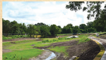
June 2017 eastward toward 2nd Street
