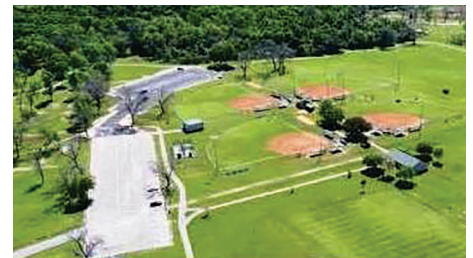
May 2017 - additional parking
